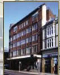
17. Fancy brick encasing structural steel. Building Society Offices, North Street. Architect: H.S. Goodhart-Rendel. 1936
