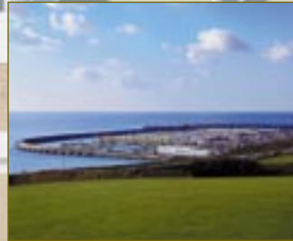
12. Reclaiming the foreshore. Brighton Marina sea wall Architect: Overton and Partners 1976
