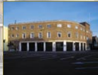
18. Traditional materials used in the Modern Manner. Fire Brigade, Preston Circus Station. Architect: Graeme Highet. 1938
